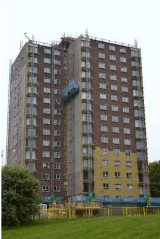
**4 June 2018,** Woodthorpe Court: Work in progress replacing the balconies, windows and outside wall insulation.
