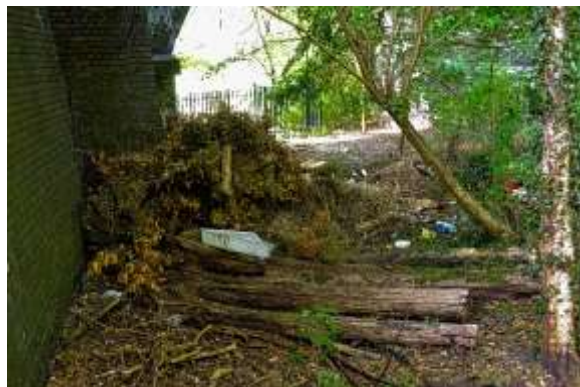
Large amounts of discarded garden waste thrown over the side of the parapet of the bridge.
