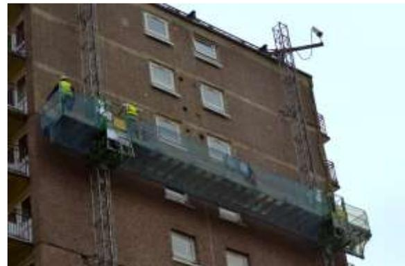
Whilst the preparation work was underway to building Extra Care Housing scheme, work was also being carried out to remove the 1960s stone cladding.
